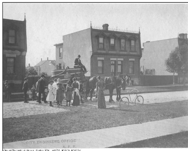
Water main repairs in 1895 meant that some areas were without water for six weeks, and water was delivered to neighbourhoods by wagon.
